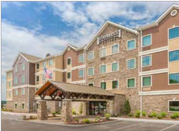
Staybridge Suites on Everhard
