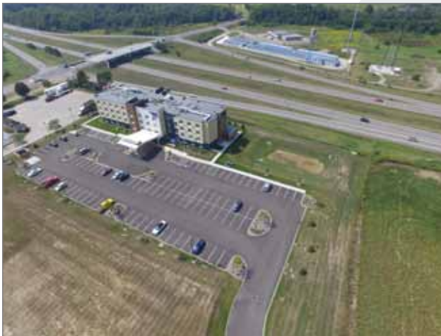
Fairfield Inn & Suites at Faircrest and I-77
